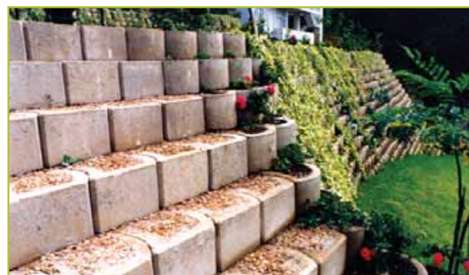
WALL AND STEPS, SMOOTH FACE FINISH
