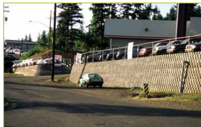
COMPOSITE WALLS IN ROUND FACE FINISH
