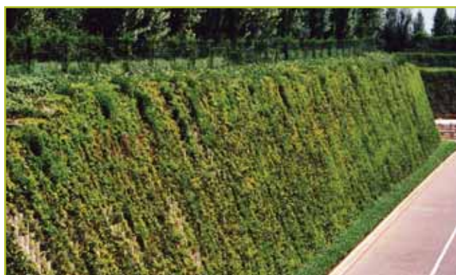
9M HIGH COMPOSITE WALL AT COMMERCIAL SITE
